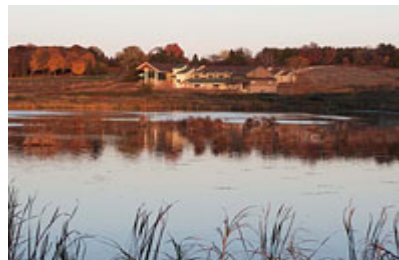
Facing across the marsh, this view showed how the building was built into the landscape and opens up to a great view of the marsh. WDNR Photo
