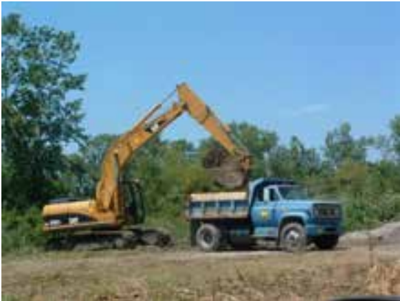
Wetland dike repair
