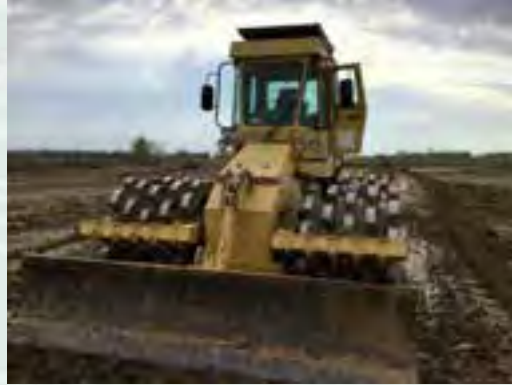
Soil Compaction & Testing
