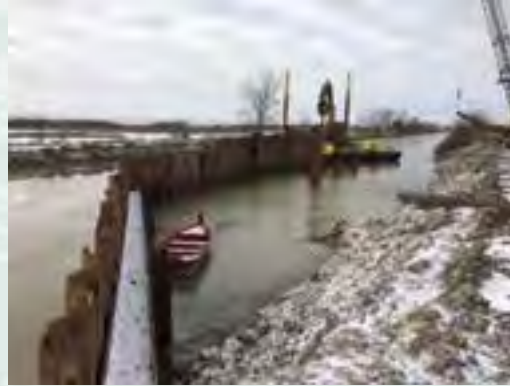
Cofferdam Installation
