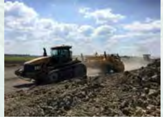
Placing Embankment
